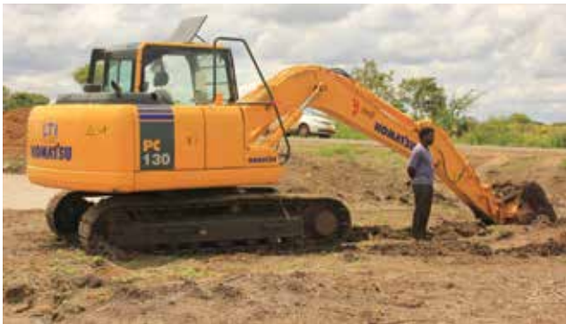
Farm Ponds Being Dug up at Hubbali
